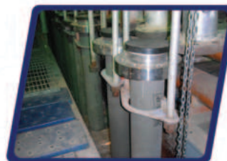
Reformer Tube Replacement
